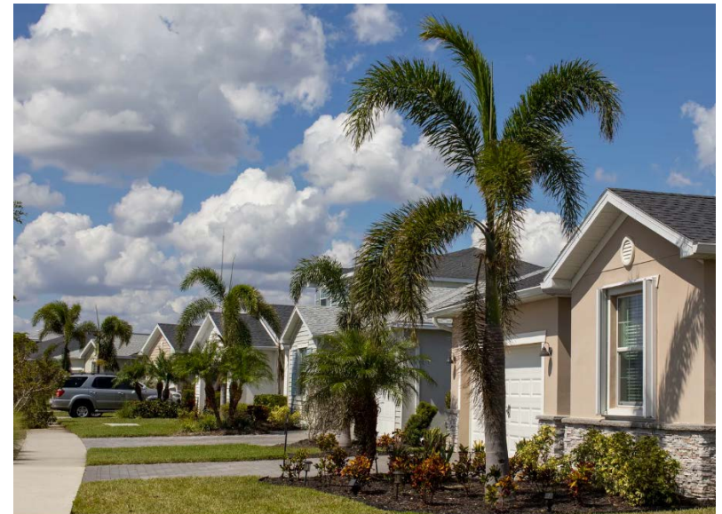
Abcock Ranch, in Florida, runs on solar power and was built to weather the worst storms. After Hurricane Ian, the community didn't lose power or water, and it experienced minimal damage. arlos Osorio for NPR
