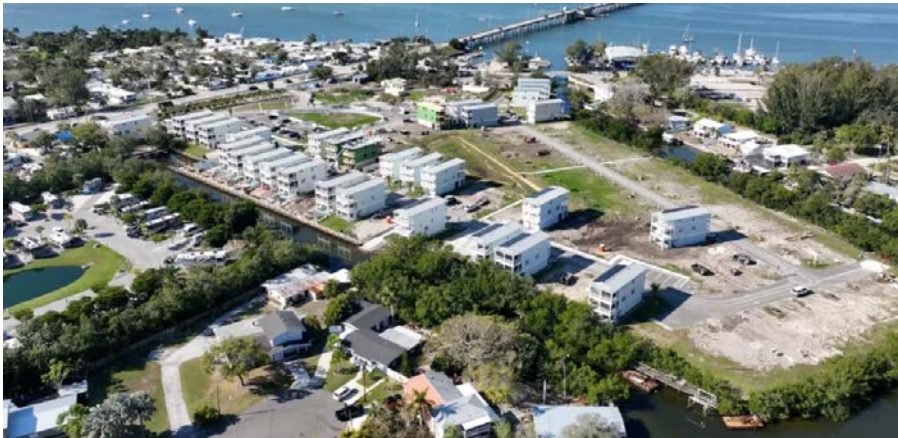
A drone image shows Hunters Point homes in Cortez, Florida, in April 2024. Billed as the first "net-zero" single-family home development in the US, Hunters Point boasts some of the most sustainable, energy-efficient and hurricane-proof homes in the country. Julian Quinones/CNN/File
